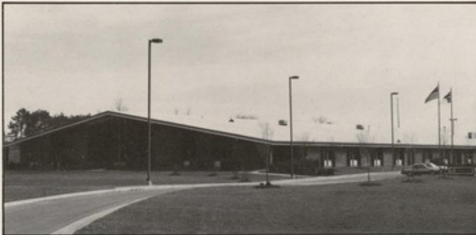
Wake County, North Carolina Plant
